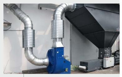
Application: Large matrix removal system for ten machines including a baler
